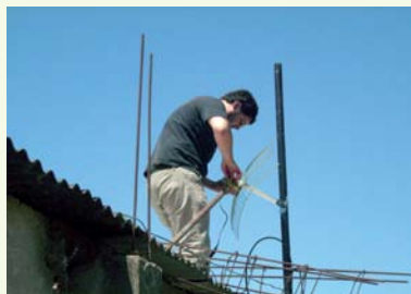
INSTALLING THE ANTENNA IN THE TOBA NEIGHBOURHOOD. PHOTO: NODO TAU
