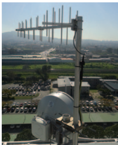
TV white space antenna transmitting broadband to local schools in Cape Town as part of the South African TVWS trial.
